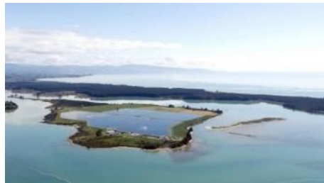
Sewage treatment at Bell Island
