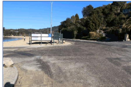
Figure 26: Kaiteriteri - Top of the Boat Ramp
