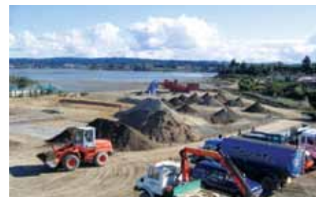
Remediation site works
